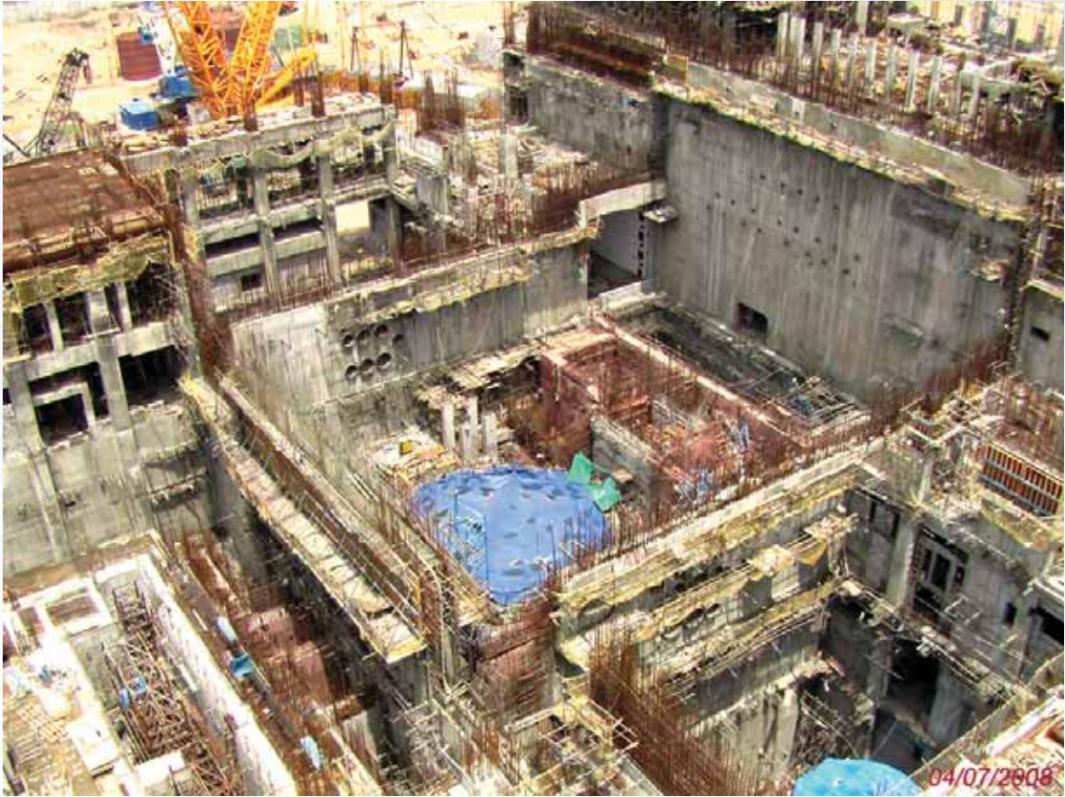
Overall view of Nuclear Island Connected Buildings (NICB)
