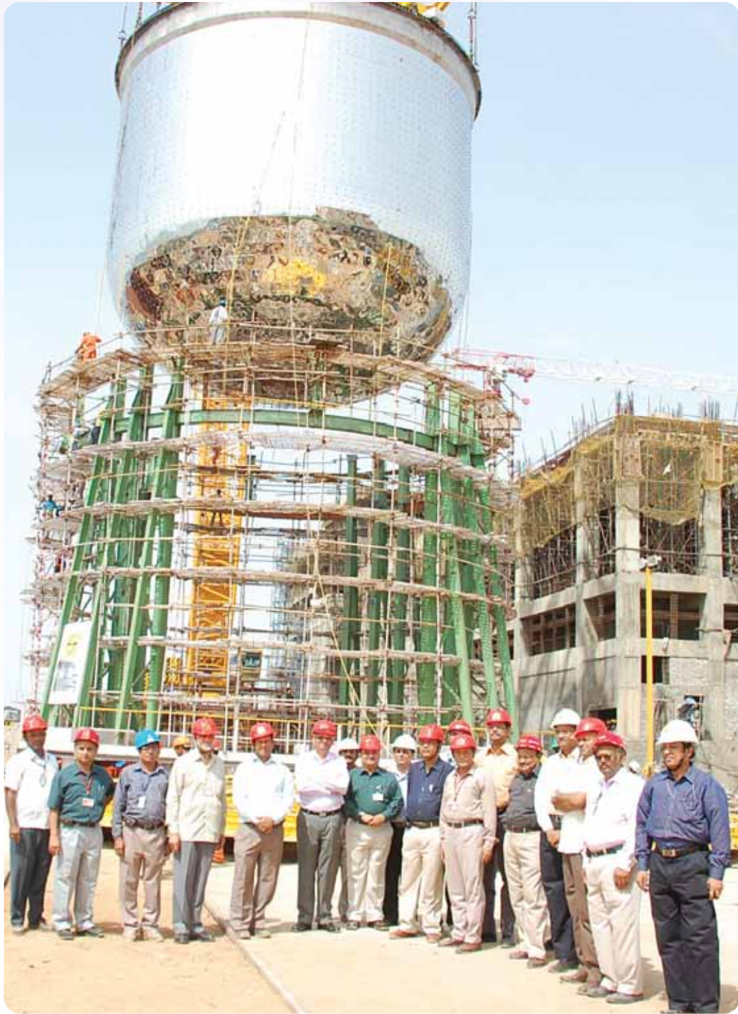
Dignitaries witnessing Safety Vessel Erection.
