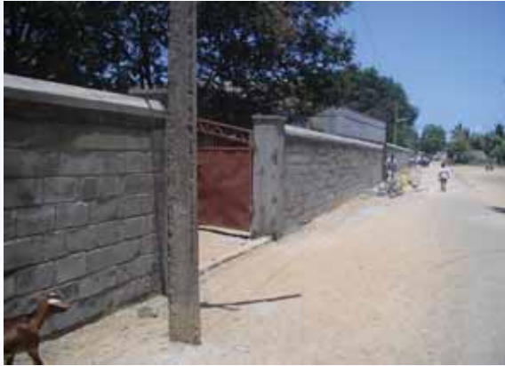
Compound Wall constructed at Neighbourhood School.
