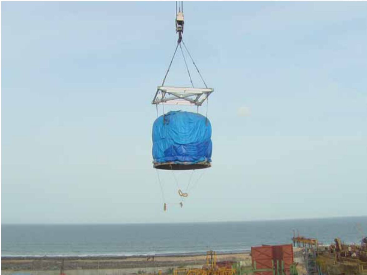
Erection of Sodium Tank
